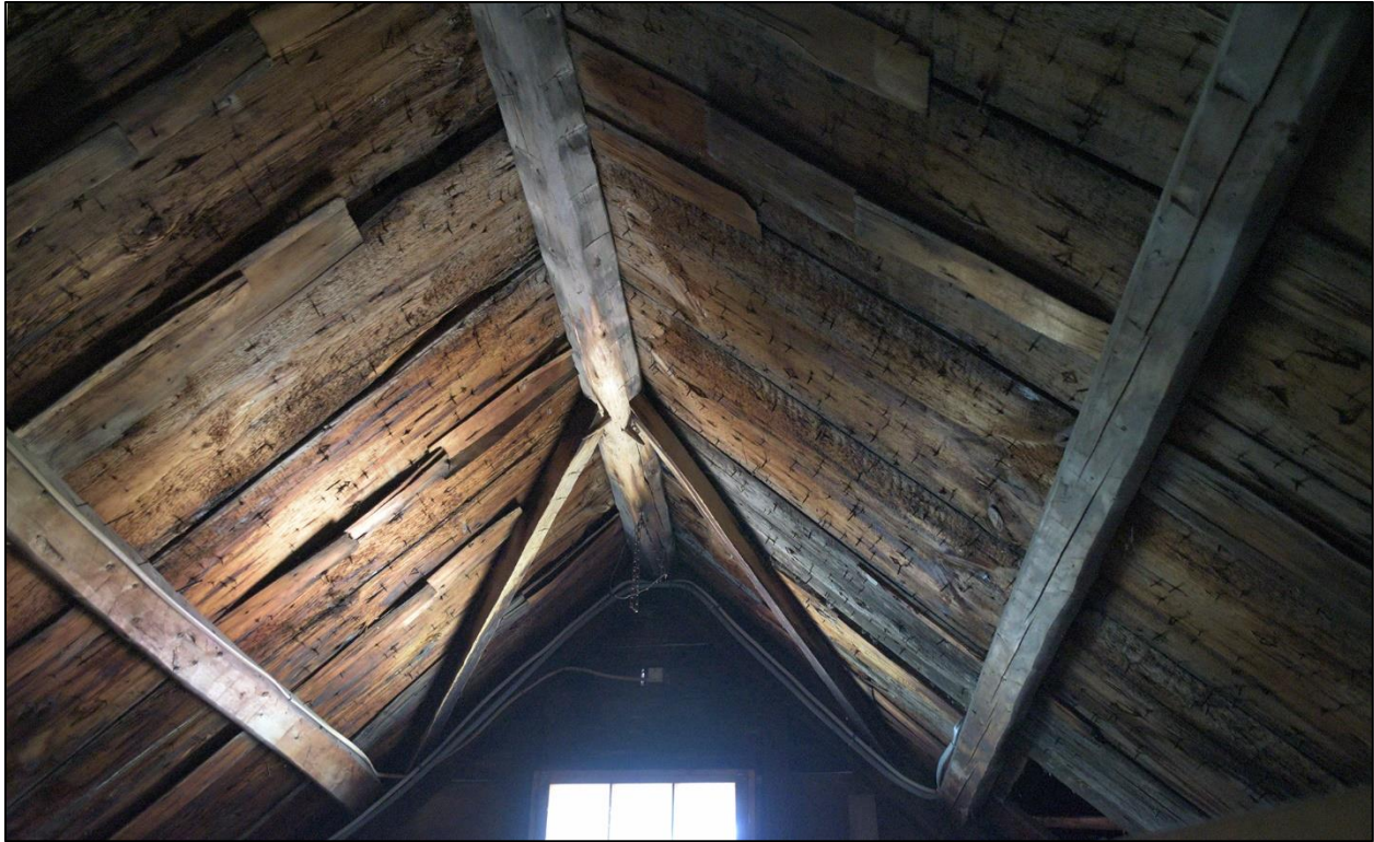
Figure 37: Attic above center chimney cape, showing roof construction (note shingles covering gaps between sheathing boards)
