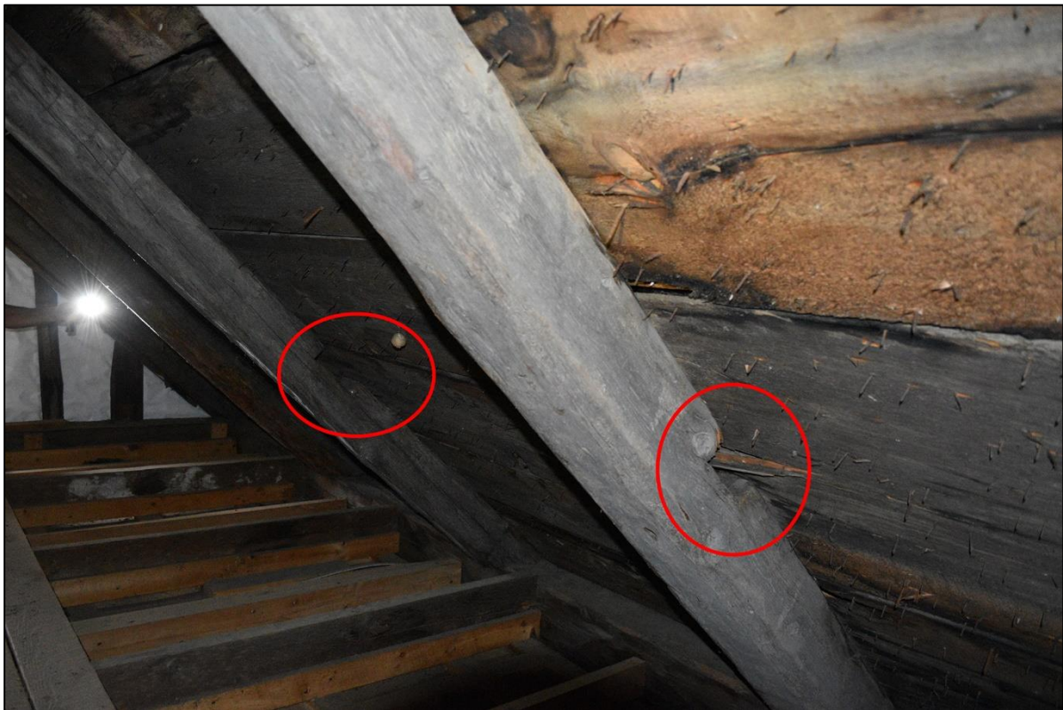
Figure 39: Empty mortises on original rafters, north ell
