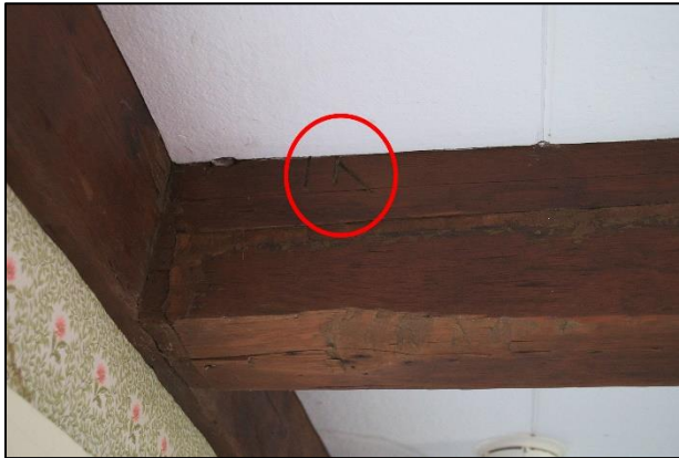
Figure 22: Roman numerals at ceiling joist
