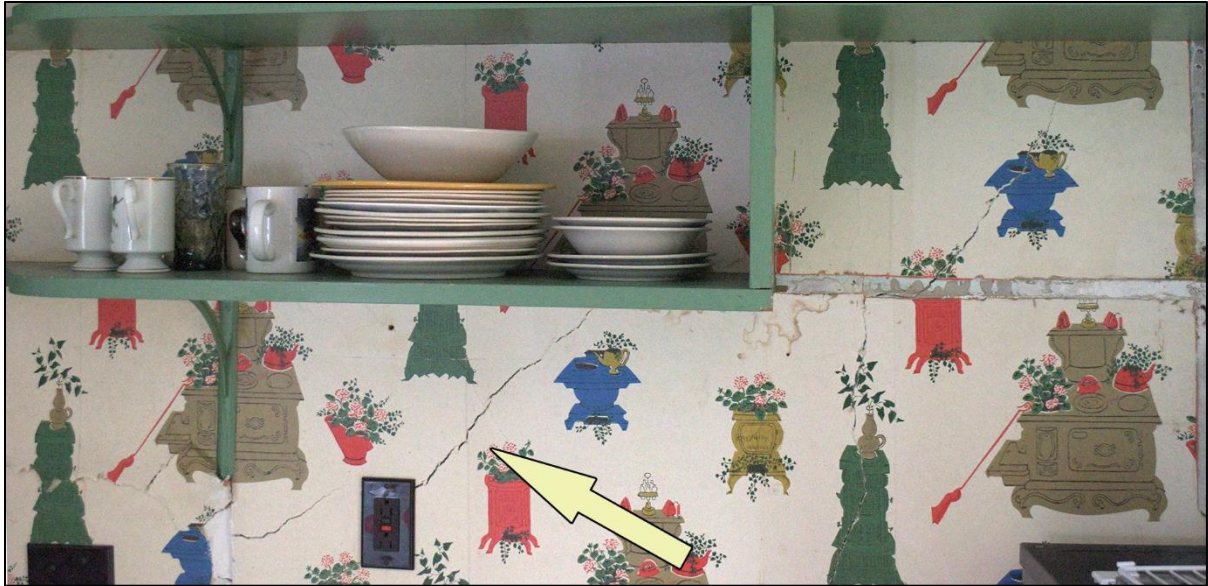
Figure 54: Plaster cracks in east wall of east wing addition (kitchen)
