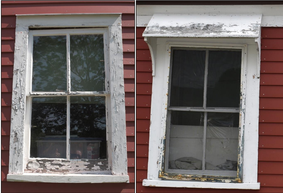
Figures 44 & 45: Typical windows showing signs of miss-alignment, cracked panes, and paint-loss
