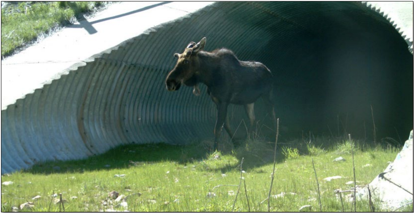
Photo 1: Moose using an under-road passage structure. Source: P. Cramer (UDOT-USU-UDWR), available from arc-solutions.org.
