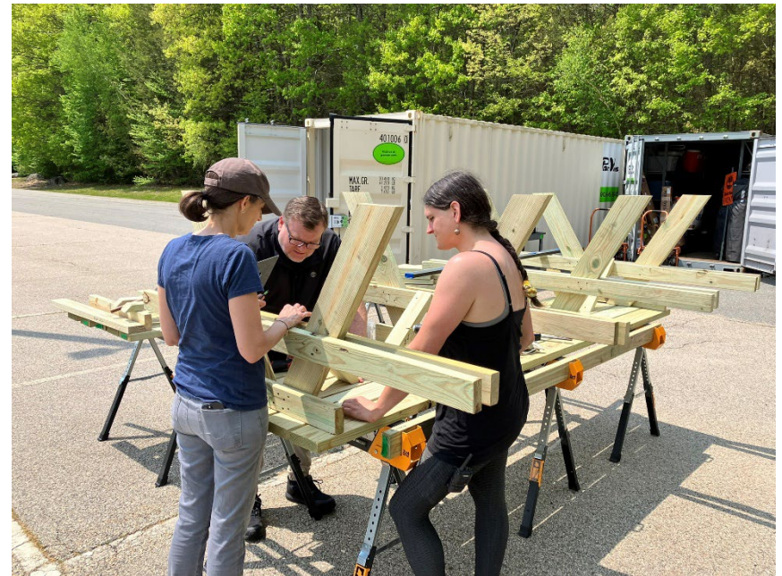
Picture 4 and 5: Bench Supports levelled and fastened
